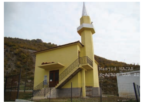
BLACK STONE in GURI-ZI, BUILT IN 2007 Serves 85 homes
