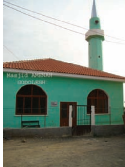
AMINA in GODOLESH, BUILT IN 2007 Serves 150 homes
