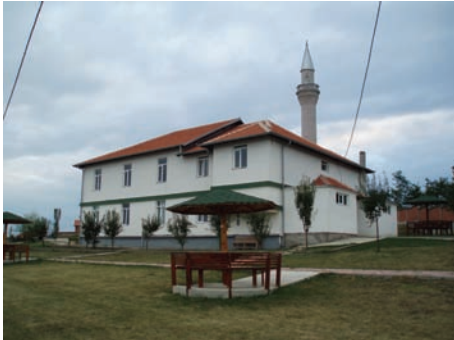
RAHMA MARINE in KOSOVO, BUILT IN 2002-2003 Serves 85 homes
