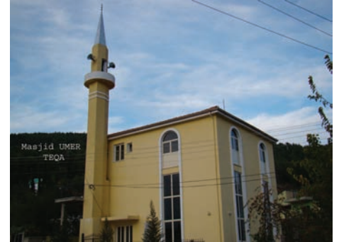
UMAR in ELBASAN, BUILT IN 2009 Serves 400 homes
